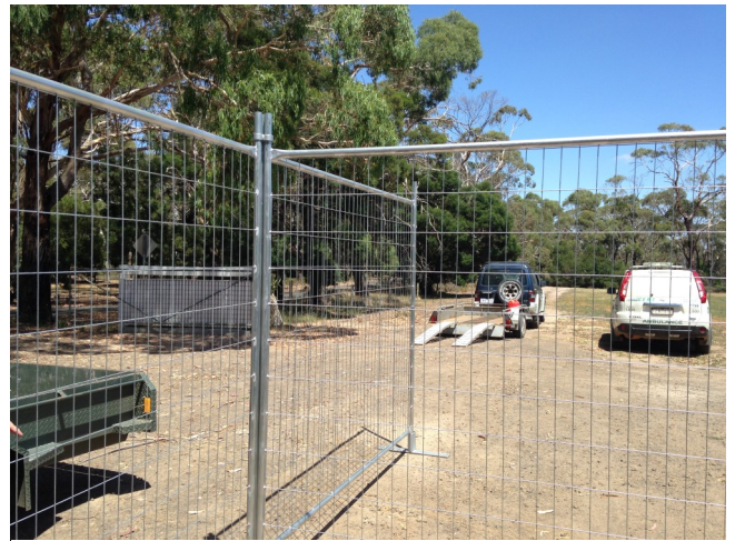
Stands can be linked together at the top for both layout flexibility and stability.
